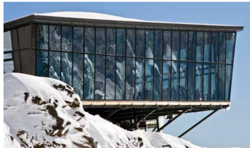
both the shed and the café were precast by Stanley Construction at their Matamata premises and transported from the Whakapapa depot by Snow Cats drawing sledges over the 2009 winter snow. The following summer LVL beams were helicoptered in and quickly erected to support the shed's upper roof structure of profiled steel cladding, which also protects the east wall. The building was completed in early 2010.
