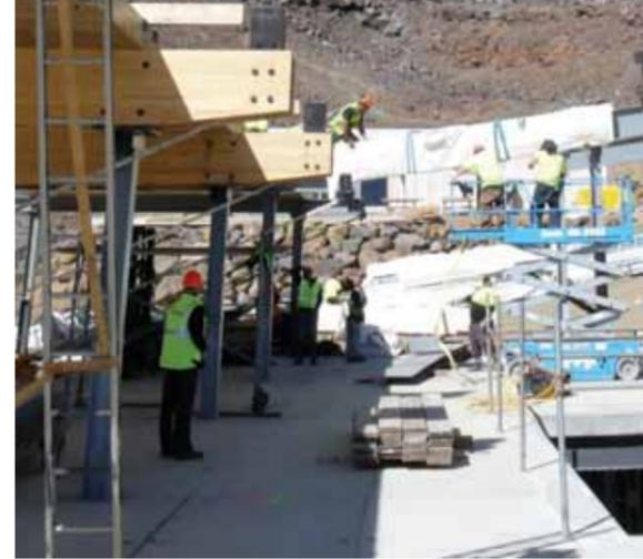
Due to helicopter weight restrictions, all the steel componentry, roof panels and structure had to be designed to weigh less than 900kgs. Precast units transported over snow were also weight-limited to loads of 1.5 tonnes – or six tonnes on a towed trailer.
