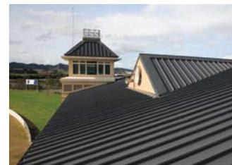
The classical lines of the building are complemented by the HiRib500 profile of the COLORSTEEL® Endura, roof which also tops off the towers. The dark roof also provides a nice contrast to the building's mostly cream-coloured exterior.
